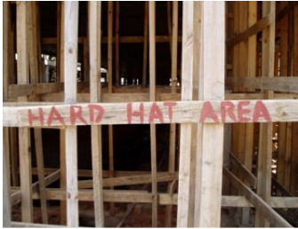
A sign at a construction site in Lusaka, Zambia
