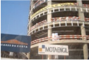
Construction site in Luanda sporting signboards of Portuguese construction companies
