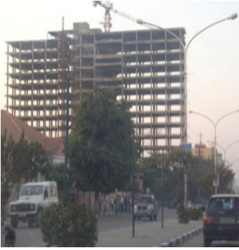
Justice palace under construction, Luanda
