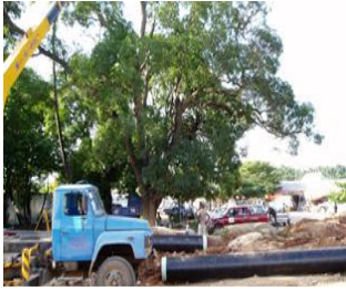
Construction site in Dar-es-Salaam, Tanzania
