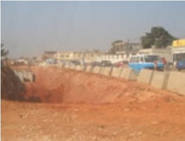
Road Rehabilitation in Luanda, Angola
