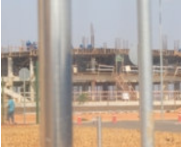
Construction at Futunga, Angola Sonangol Project
