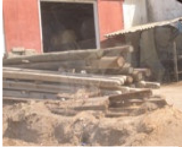
Construction site in Luanda, Angola
