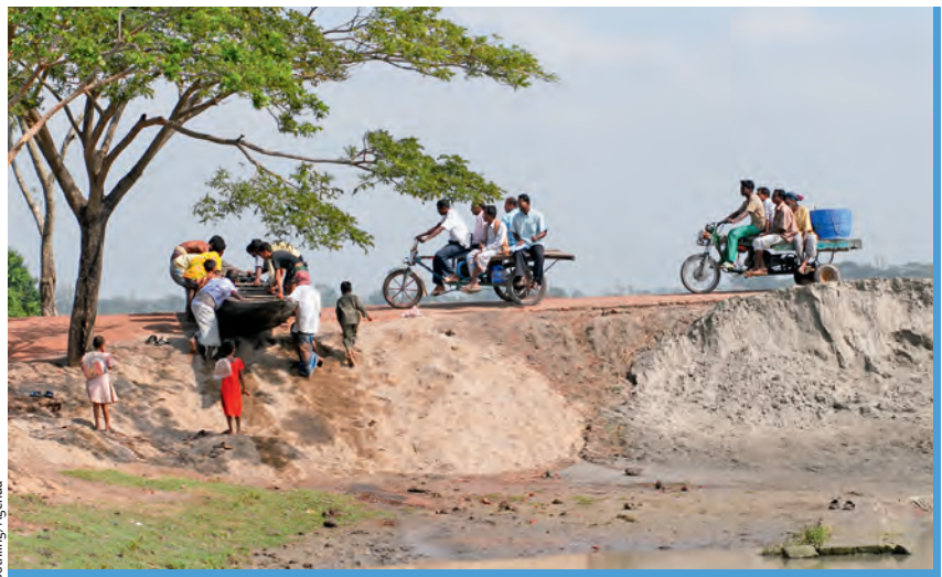
Roads are built on levees and serve flood protection purposes too.
