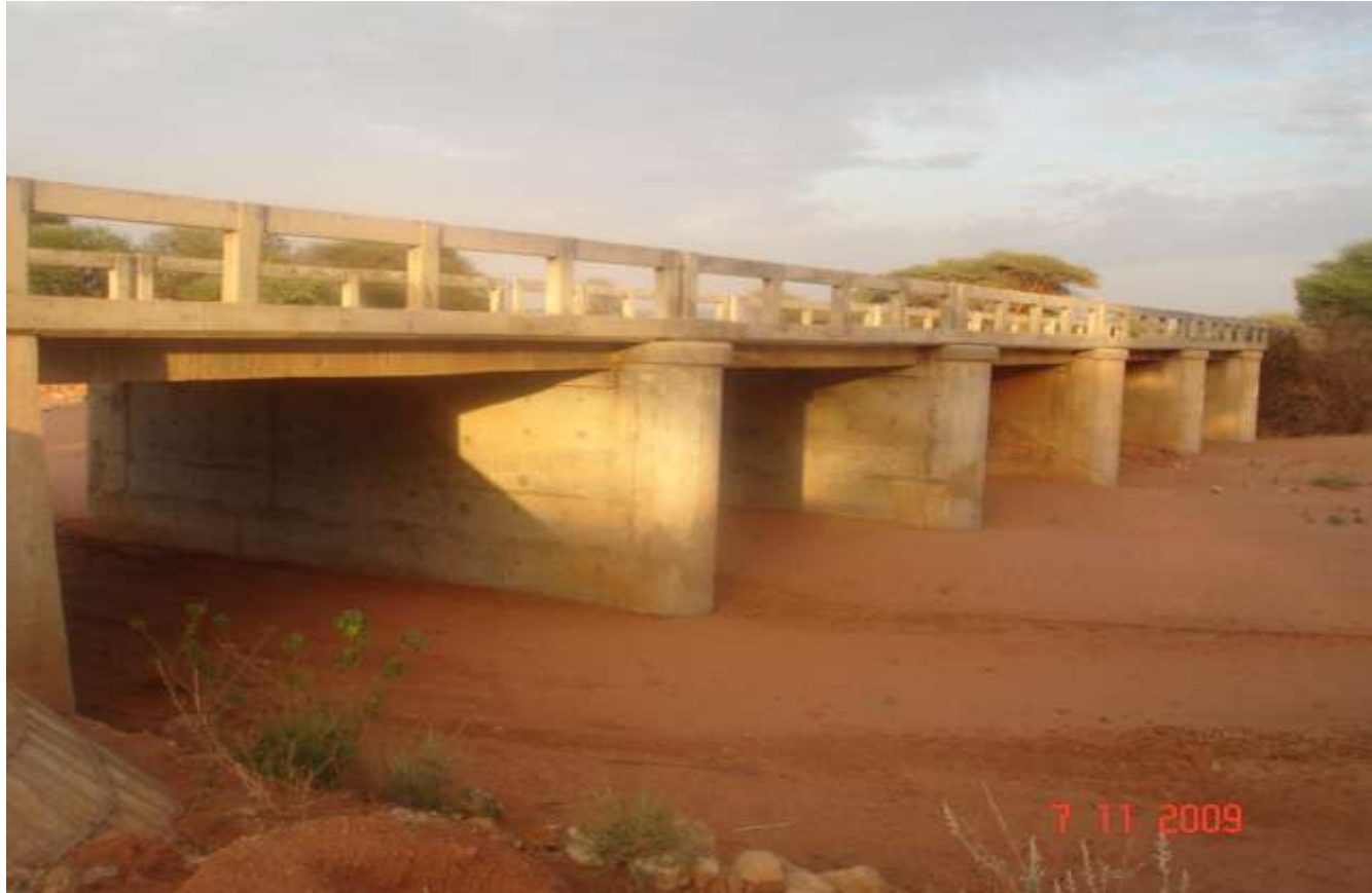
Reconstruction of Bridges
