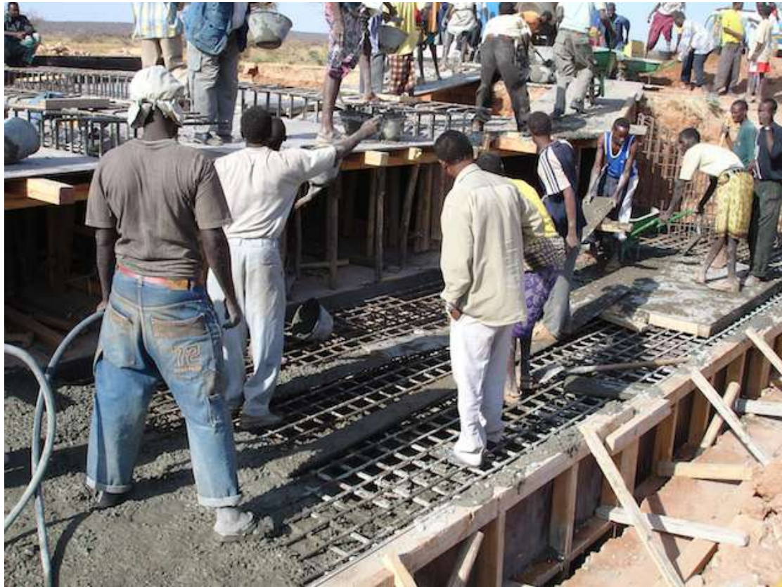
Reconstruction of culverts
