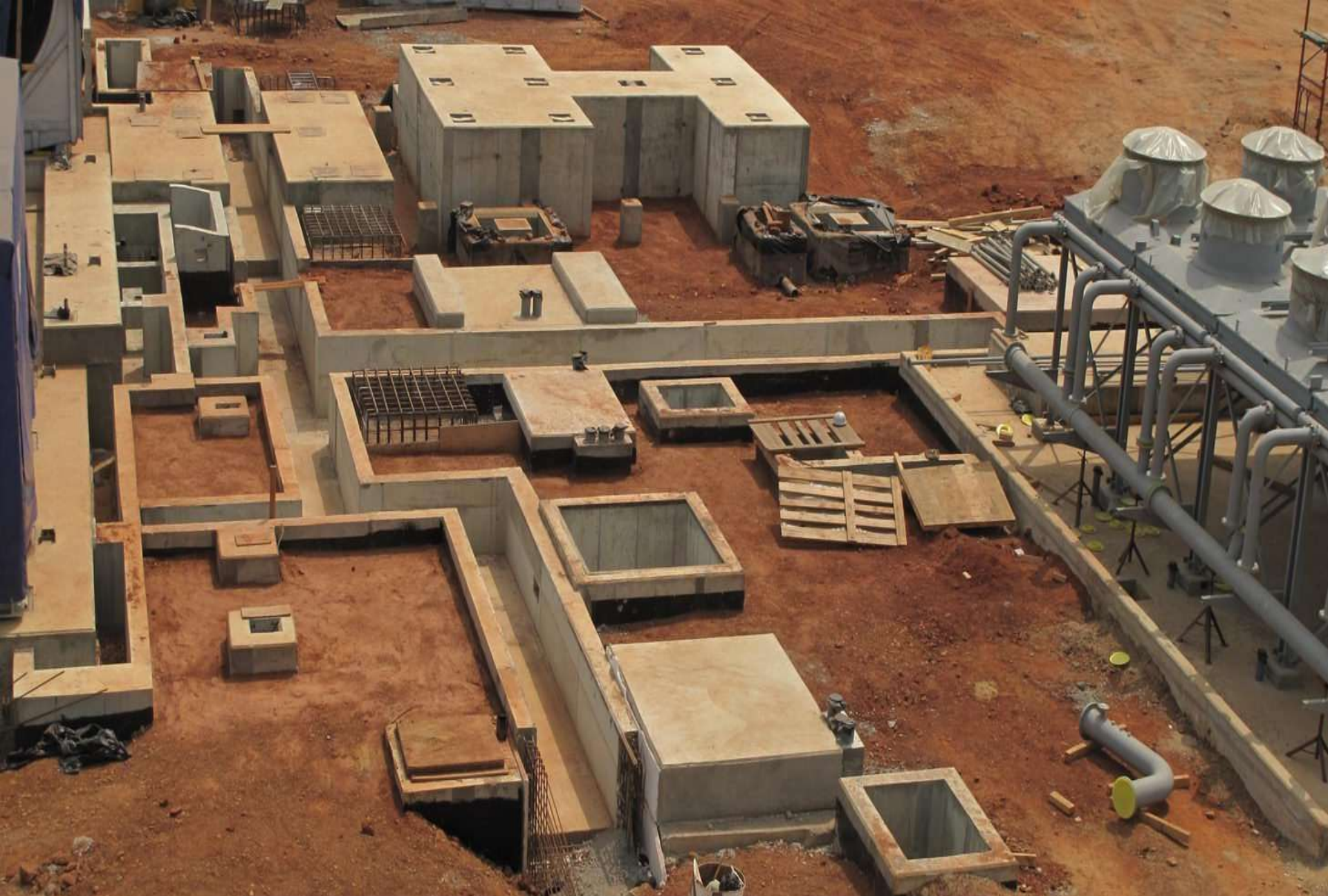
ALL SOUTH SIDE CIVIL WORKS COMPLETE - JAN 02, 2009
